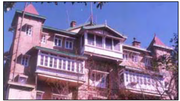
Facade of Rani Amrit Kaur Building
