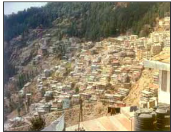
Constructions without Proper Roads at Sanjauli
