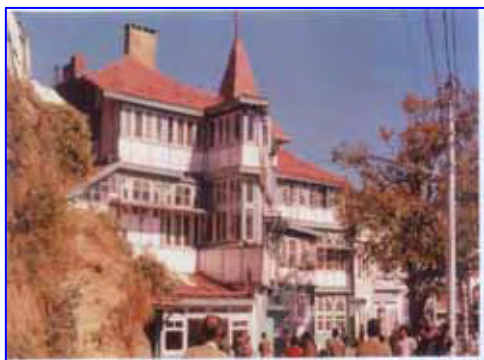
Telephone Exchange Building
