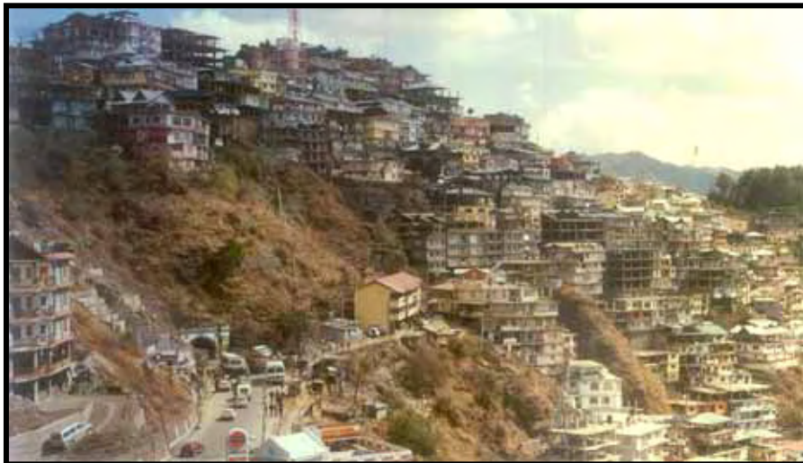
Massive Construction at Cemetery without Proper Accesses
