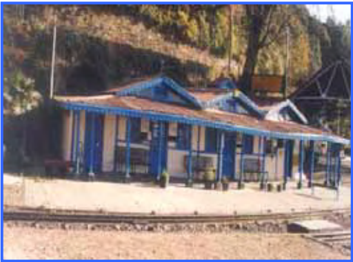
Kalka-Shimla Rail Line
