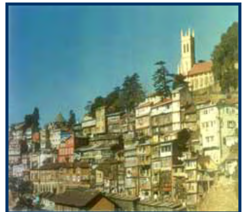
Obsolete Construction in Heritage Zone Near Ridge Crying for Re-Modelling
