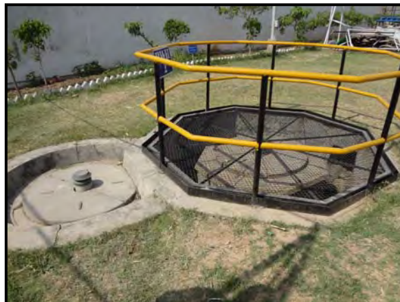
Fig 12.62 Rain water harvesting tank - Underground
