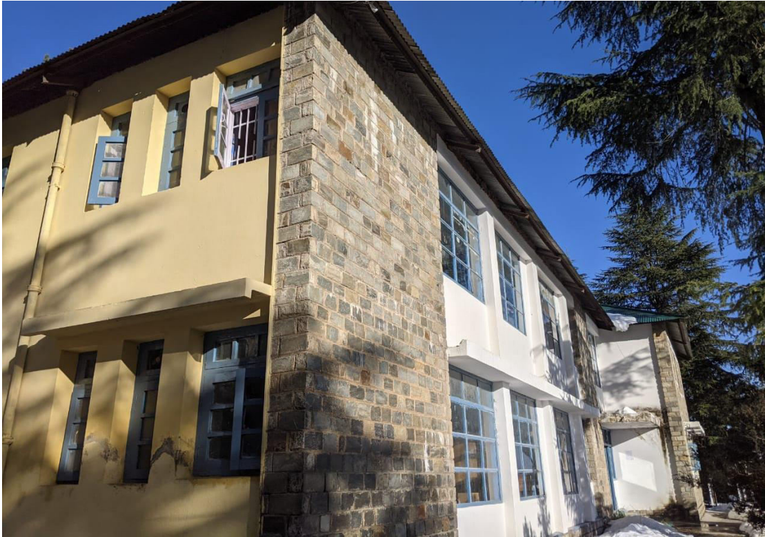
Figure 8.1- Load Bearing Structure in Government accommodation
