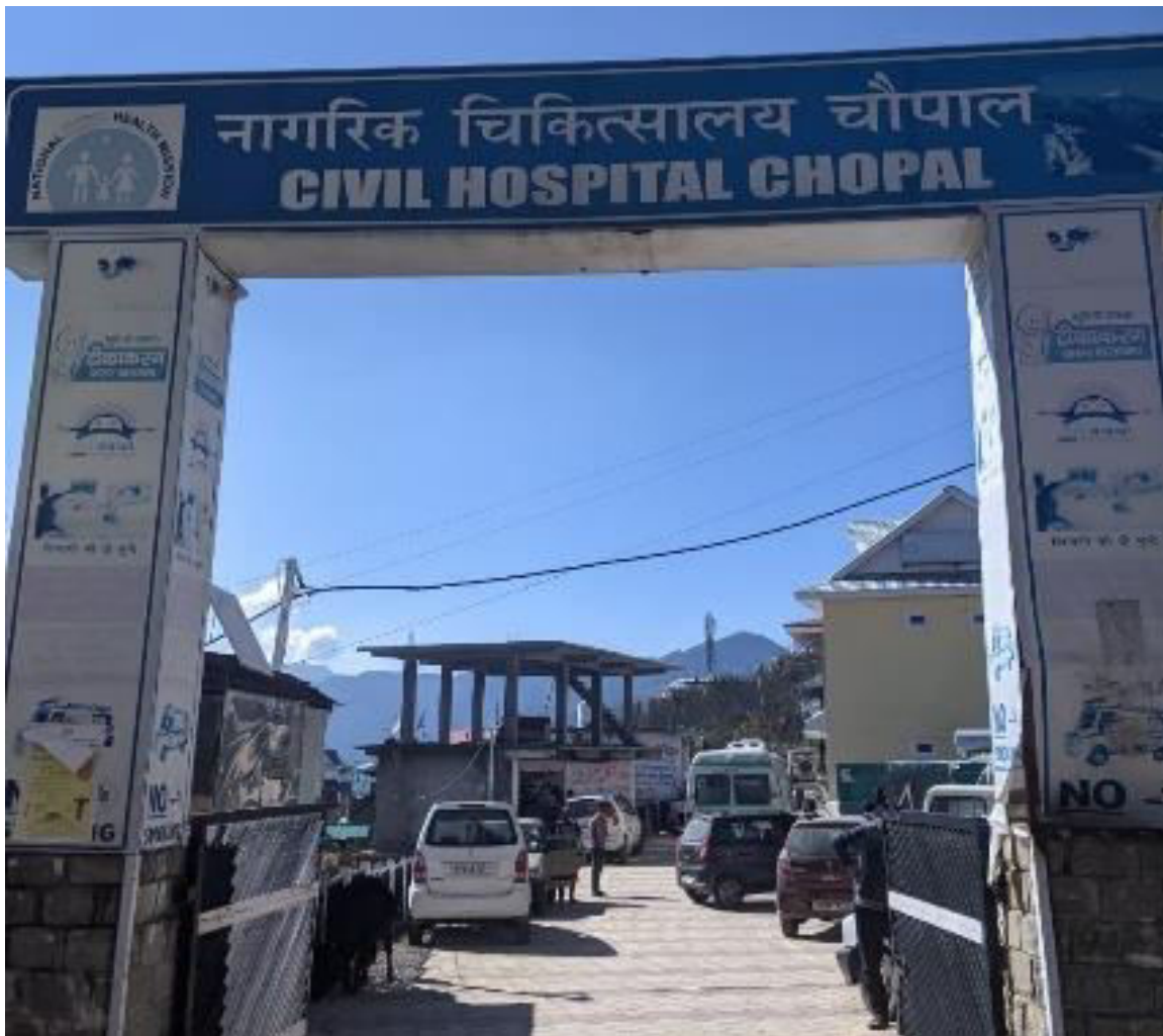
Figure 6.7- Civil Hospital Chopal
