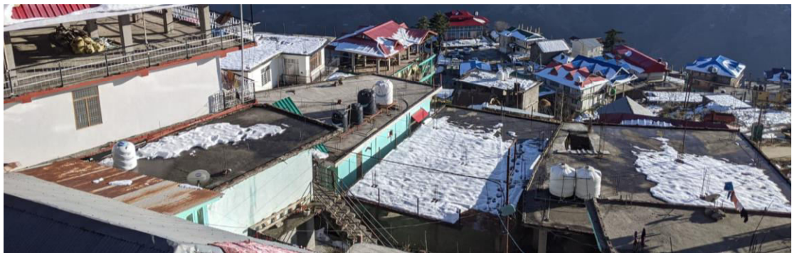
Figure 4.1- Set-back violations in Chopal
