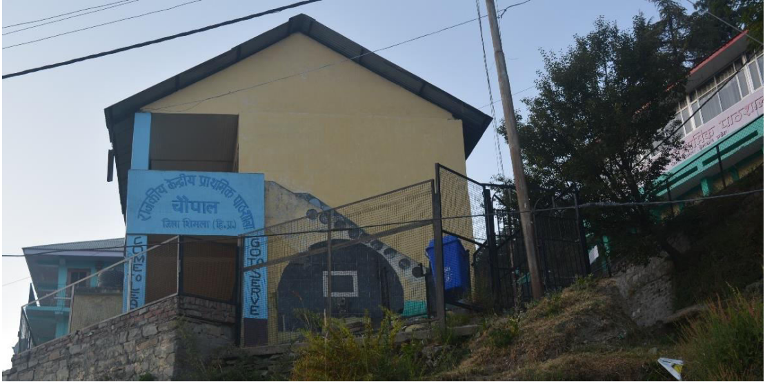
Figure 6.5- Govt. Central Primary School
