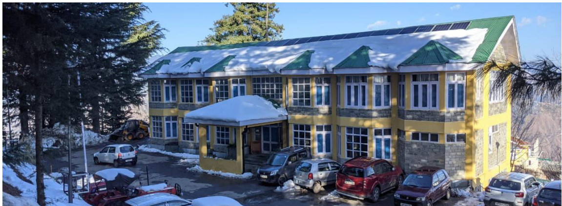
Figure 5.11- PWD Rest House Chopal
